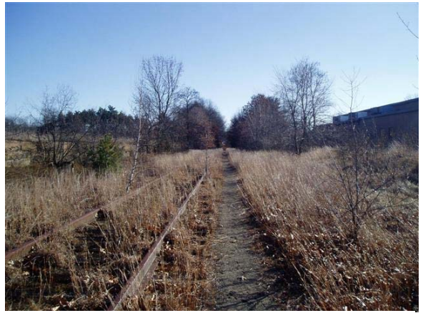
Figure 2: Corridor Between Commonwealth Avenue and Bridge No. 14.81
