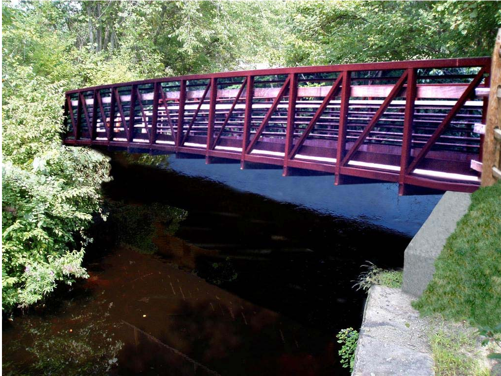
Figure 43: Alternative 3 - Prefabricated Bridge
