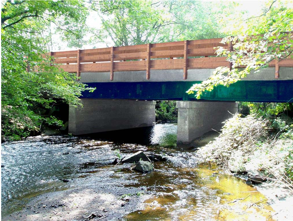
Figure 45: Alternative 1 - Reuse of Existing Bridge Structure
