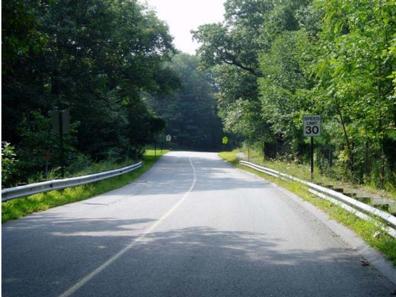
Figure 32: Looking West Along Powder Mill Road (Above Rail Corridor)
