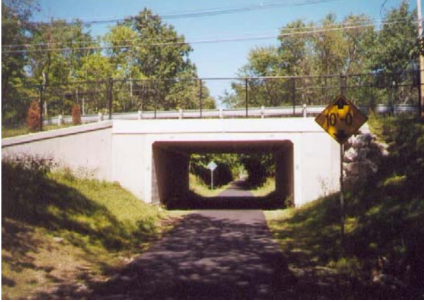
Figure 39: Concrete Box Culvert Along the Nashua River Rail Trail
