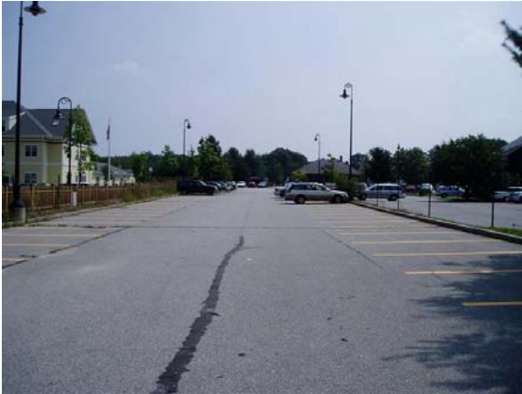
Figure 34: MBTA Commuter Parking Lot Looking South Along Rail Corridor
