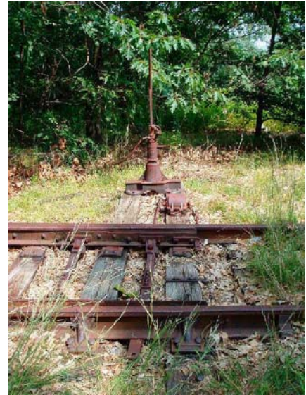
Figure 56: Track Switch at Spur Line
