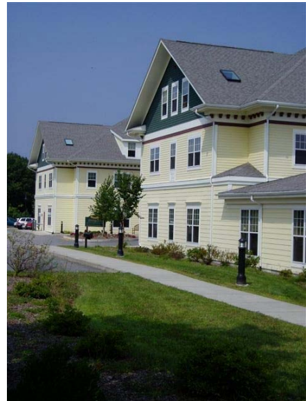
Figure 8: Concord Park Facility on East Side of Rail Corridor
