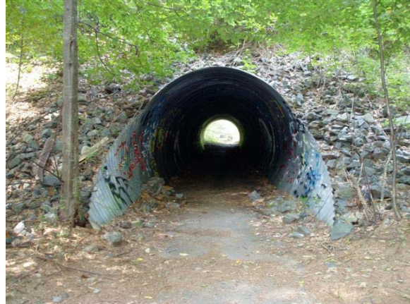
Figure 33: Existing Corrugated Metal Pipe Underpass
