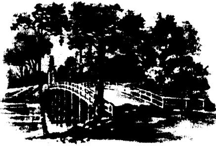
OLD NORTH BRIDGE
