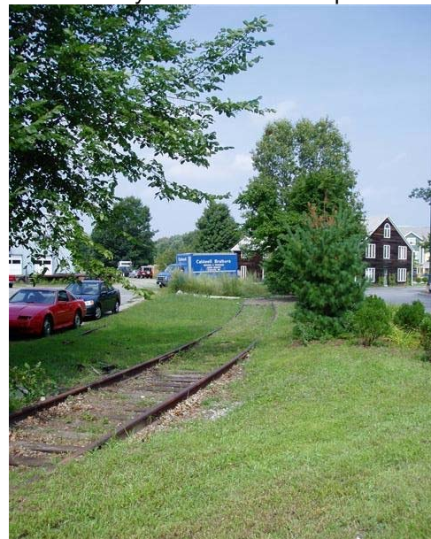
Figure 36: Looking South Along Spur Track
