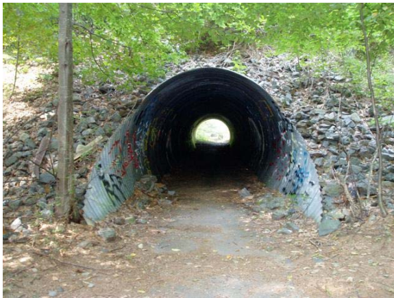
Figure 37: Existing Corrugated Metal Pipe Underpass
