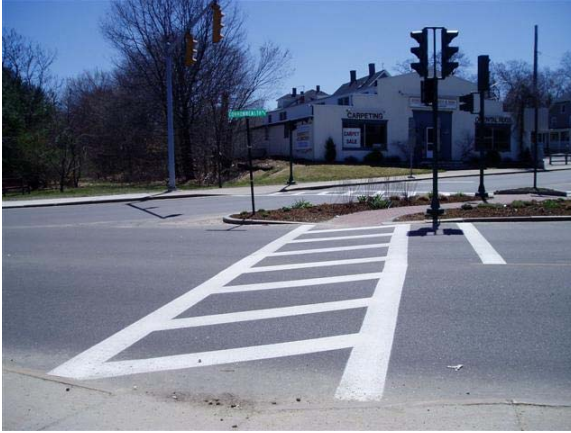
Figure 26: Pedestrian Crossing #1 Commonwealth Avenue at Main Street (Route 62)
