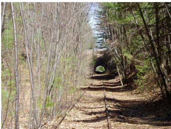
Figure 38: Looking North Along the Corridor
