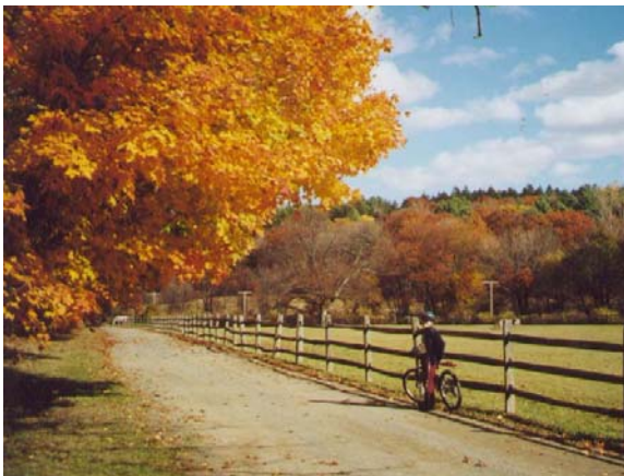
Figure 50: Post and Rail Fence to Separate Rail Trail from Adjacent Private Land
