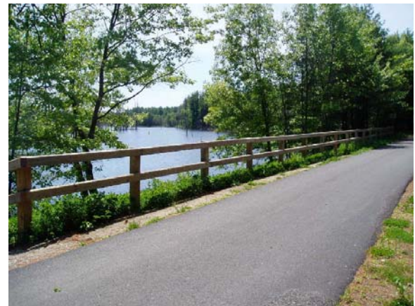
Figure 51: Wood Rail Fence to Discourage Users from Leaving the Trail
