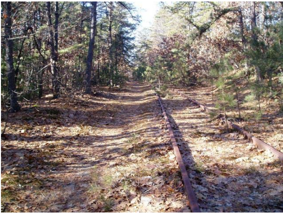
Figure 1: Corridor Between Bridge No. 13.86 and Commonwealth Avenue
