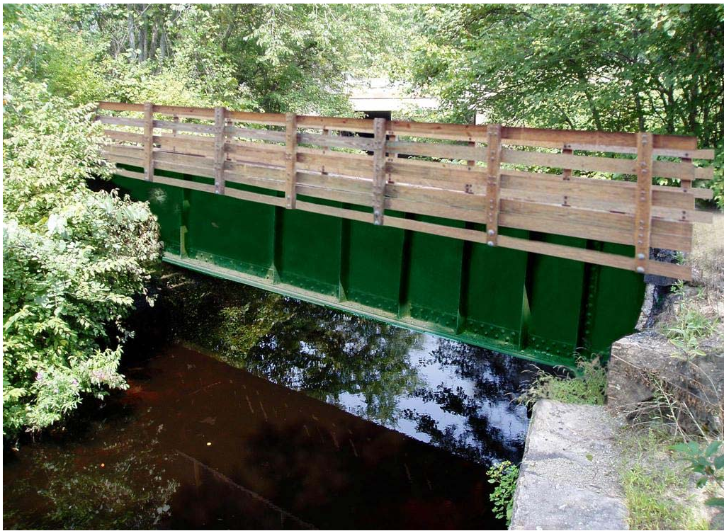
Figure 41: Alternative 1 - Reuse of Existing Bridge Structure
