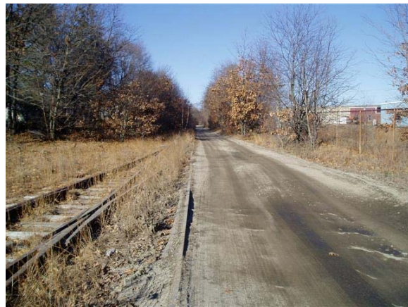
Figure 10: MCI-Concord Access Drive Along Corridor
